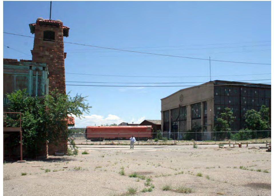
Southwest Corner showing proximity to Tank Shop in background.
