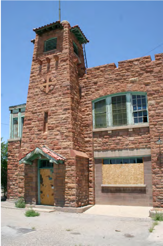
Firehouse, South Elevation - Detail.
