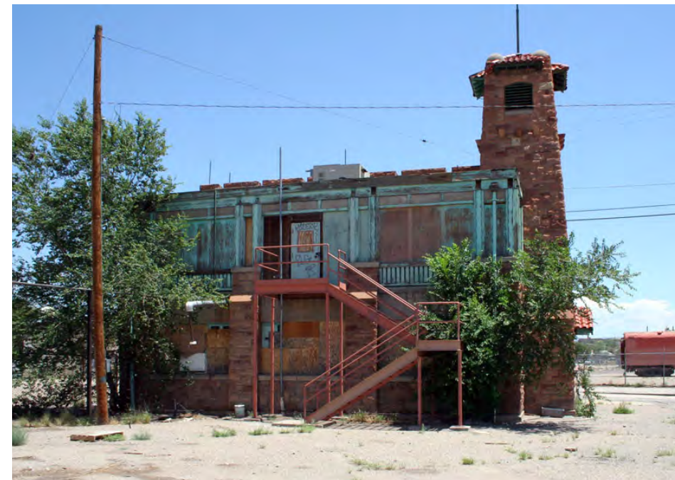
Firehouse, West Elevation.
