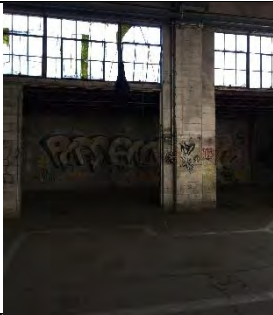
Figure 3 Interior of Fine Shop
