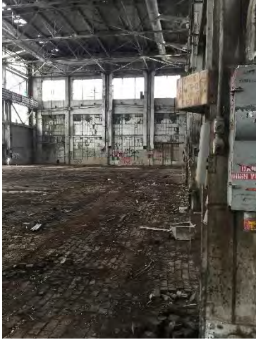
Figure 1 Interior of Boiler Shop
