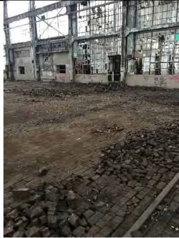
Figure 4 Interior of Boiler Shop
