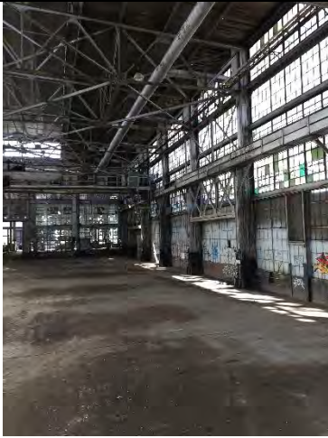
Figure 1 Interior of Tender Repair
