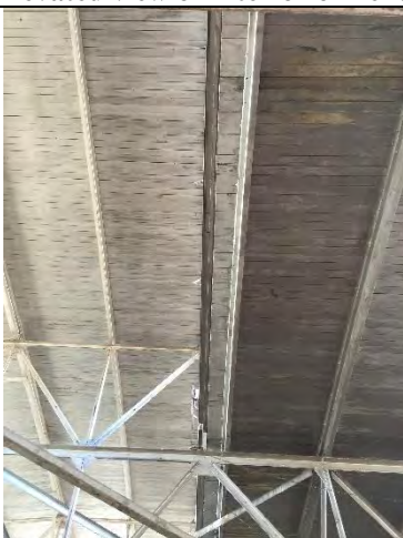
Figure 5 Interior ceiling of Tender Repair
