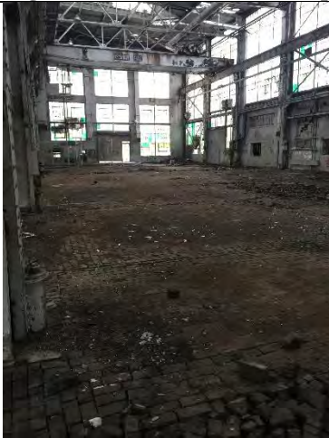
Figure 5 Interior of Boiler Shop
