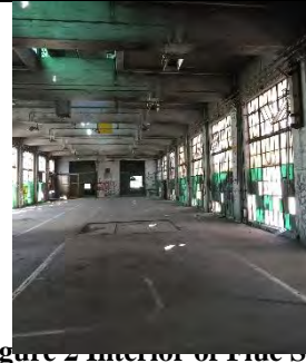
Figure 2 Interior of Fine Shop
