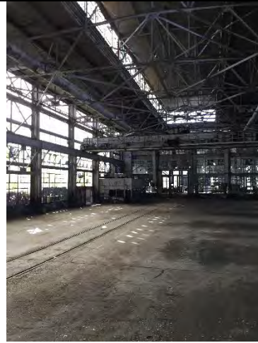
Figure 2 Interior of Tender Repair
