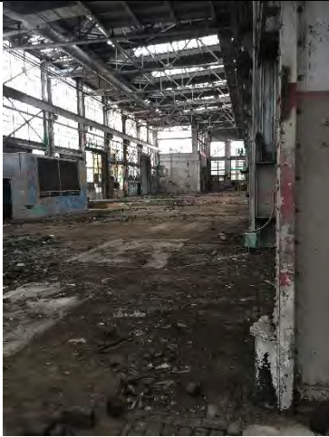
Figure 3 Interior of Boiler Shop
