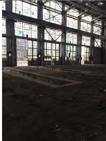
Figure 6 Interior of Boiler Shop
