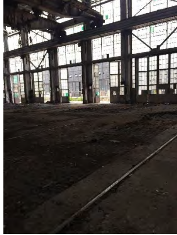
Figure 2 Interior of Boiler Shop
