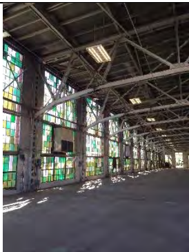
Figure 3: Interior of Blacksmith Shop
