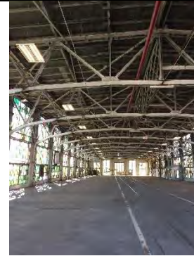
Figure 2: Interior of Blacksmith Shop
