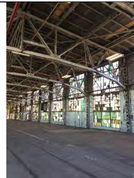
Figure 4: Interior of Blacksmith Shop
