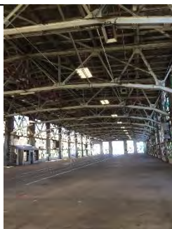
Figure 5: Interior of Blacksmith Shop
