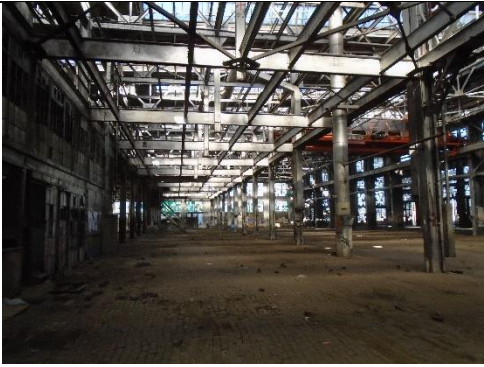
Figure 3 Interior of Machine Shop
