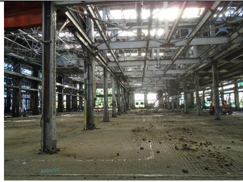
Figure 4 Interior of Machine Shop
