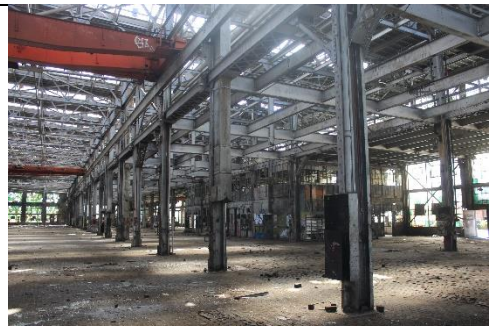
Figure 6 Interior of Machine Shop
