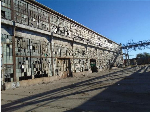
Figure 1 Exterior of Machine Shop
