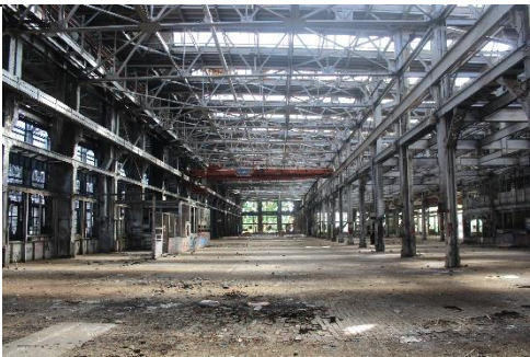
Figure 5 Interior of Machine Shop
