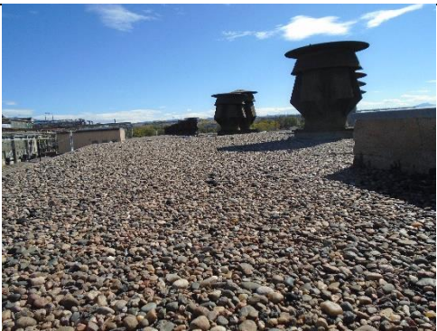
Figure 5 Roof of Welding Shop
