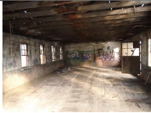
Figure 4 Interior of South Wash Room
