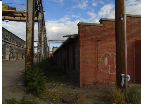
Figure 2 Exterior of South Wash Room
