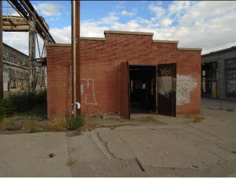
Figure 1 Front Exterior of South Wash Room
