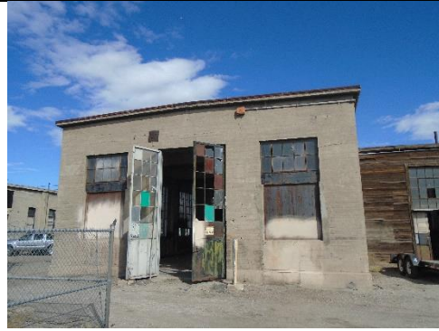
Figure 2 Back of Babbitt & Welding Shop
