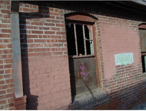
Figure 3 Window Exterior of South Wash Room
