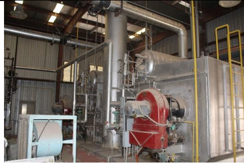
Figure 4 Interior of Power House
