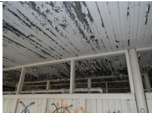
Figure 6 Interior of South Wash Room
