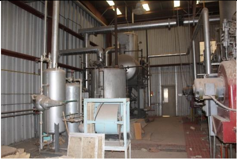
Figure 3 Interior of Power House
