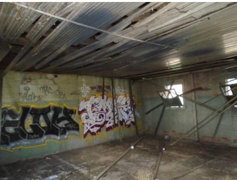
Figure 5 Interior of South Wash Room
