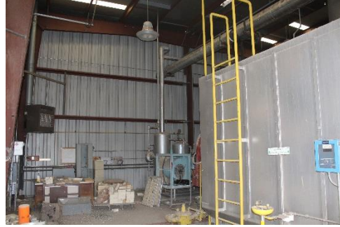
Figure 2 Interior of Power House
