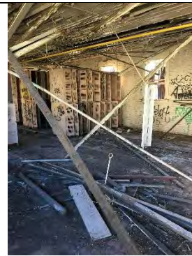
Figure 4 Interior of North Wash Room
