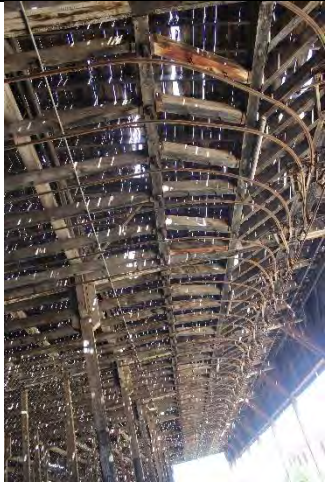
Figure 1, Open Side of Sheet Metal House
