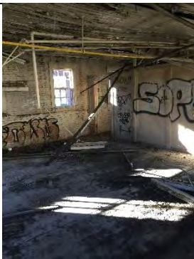
Figure 5 Interior of North Wash Room
