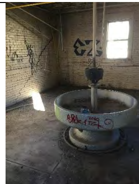
Figure 6 Interior of North Wash Room
