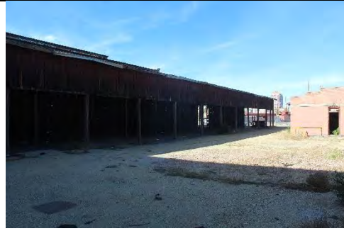
Figure 2, Sheet Metal House, East Side
