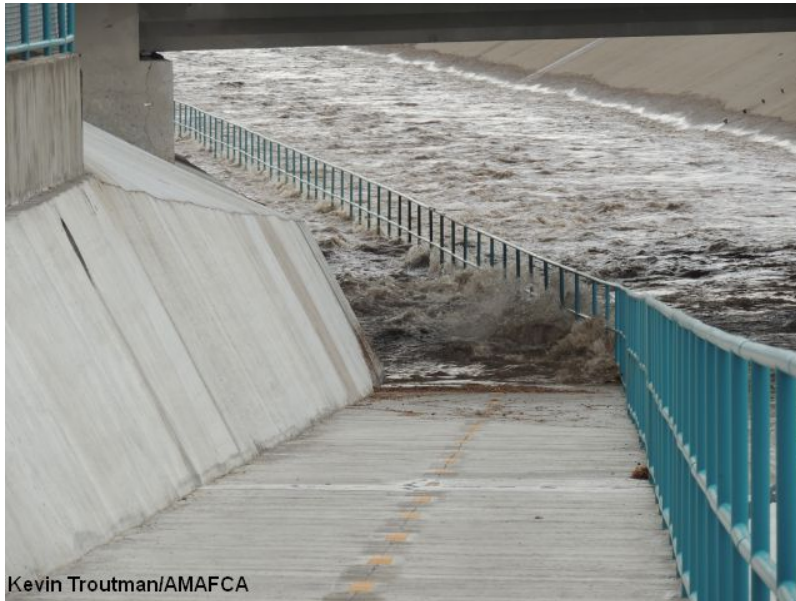
Figure 4.4: Flooding along the Osuna Bike Notch on July 26 th , 2013
