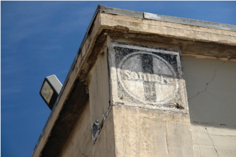
Cast-in-place concrete structure of Storehouse Building with painted logo
