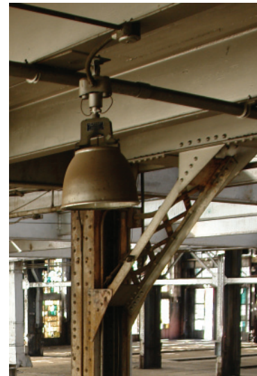
Machine Shop, Existing High Bay Lighting
