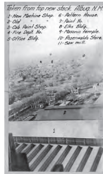
View from atop SMOKESTACK
