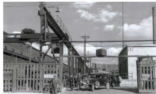
Historic Rail Yards Entrance
