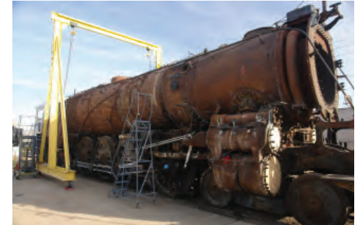
ATSF 2926 Restoration, Albuquerque, NM
