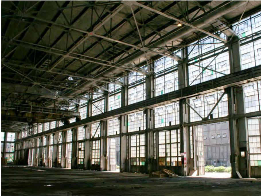
*Boiler Shop, Erecting Bay, Fully Glazed southern elevation with 18' tall operable doors.*
