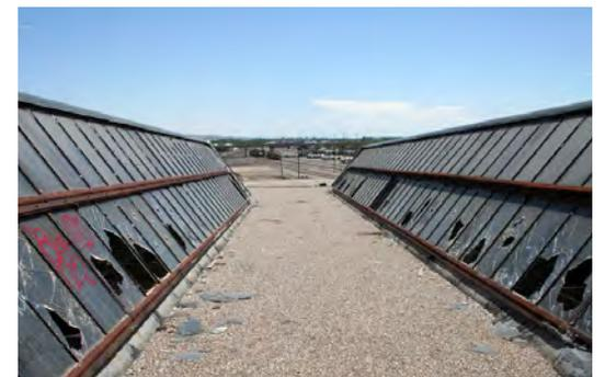
*Built-up roofing, positive slope to South.*
