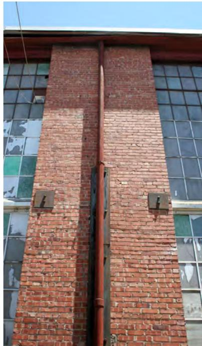
West/East Elevation, Steel Plate upgrades.
