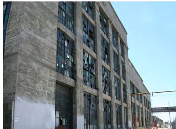
West Elevation, Cast in Place Concrete Frame.
