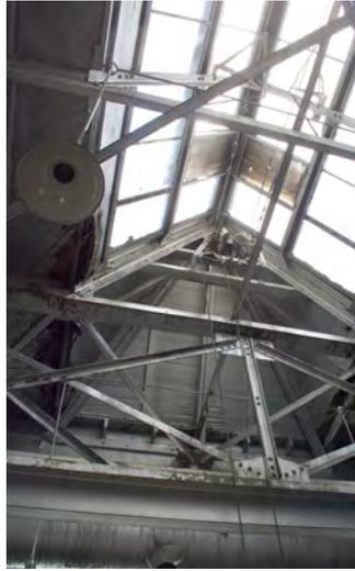
Gear/Pulley mechanism for skylight operation.
