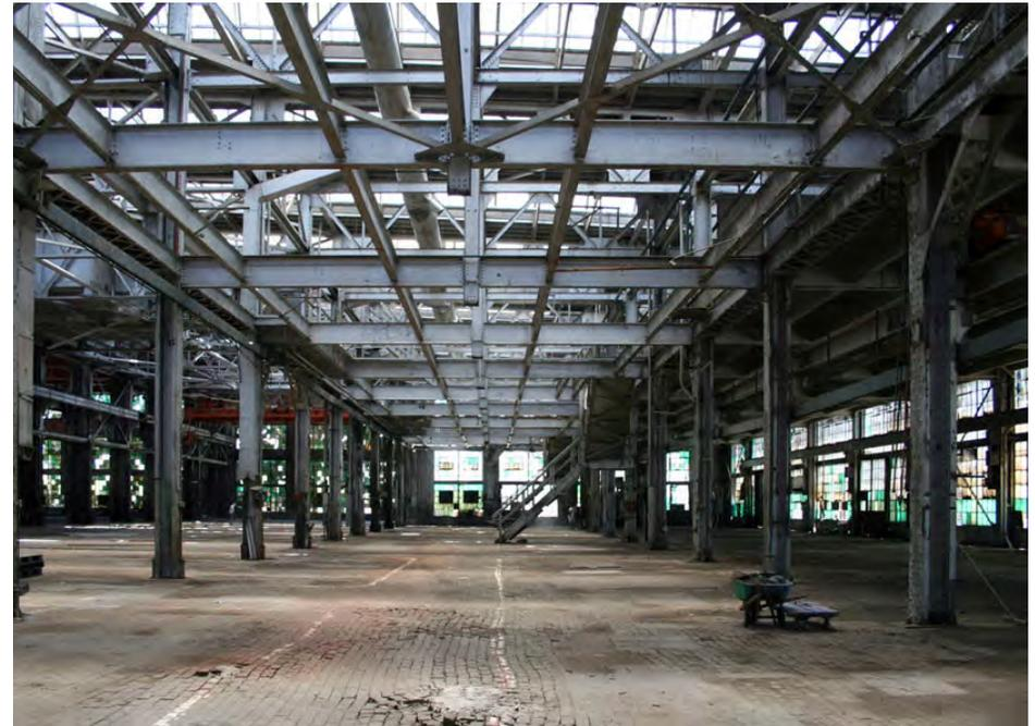
*Machine Shop, Light Machinery Bay, Pyramidal skylights run between the Heavy and Light Machinery Bays*
