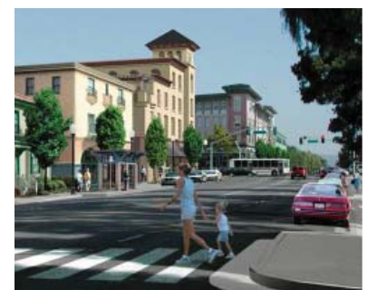
Curb extension at intersection
