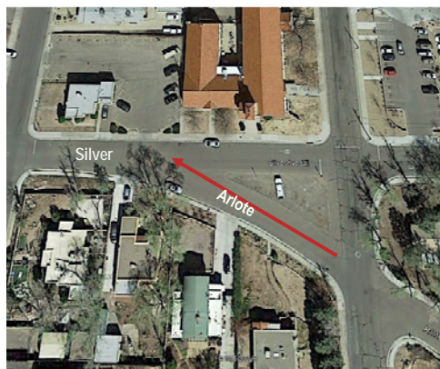
Existing Silver/Arlote intersection
