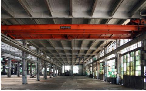
Machine Shop, Bay #1 - Below board formed, cast in place, concrete mezzanine.
