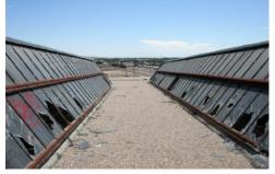
Built-up roofing, positive slope to South.
