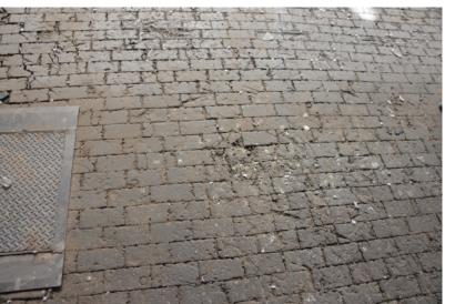
Machine Shop Floor, 3" thick Kreolite creosoted woods blocks sit on a 6" thick concrete floor to dampen sound
