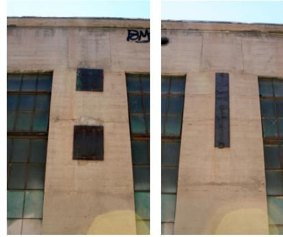
Steel plate seismic upgrades
