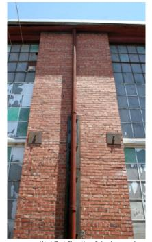
West/East Elevation, Seismic upgrades.
