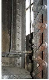
Crank mechanism for skylight operation.
