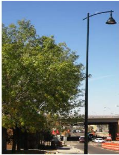
New lighting on Coal Avenue
