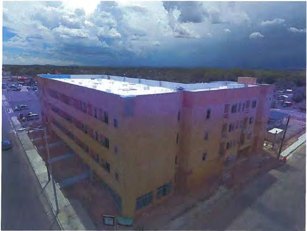
Under Construction—76 units in two phases, commercial on the ground floor, residential on top
