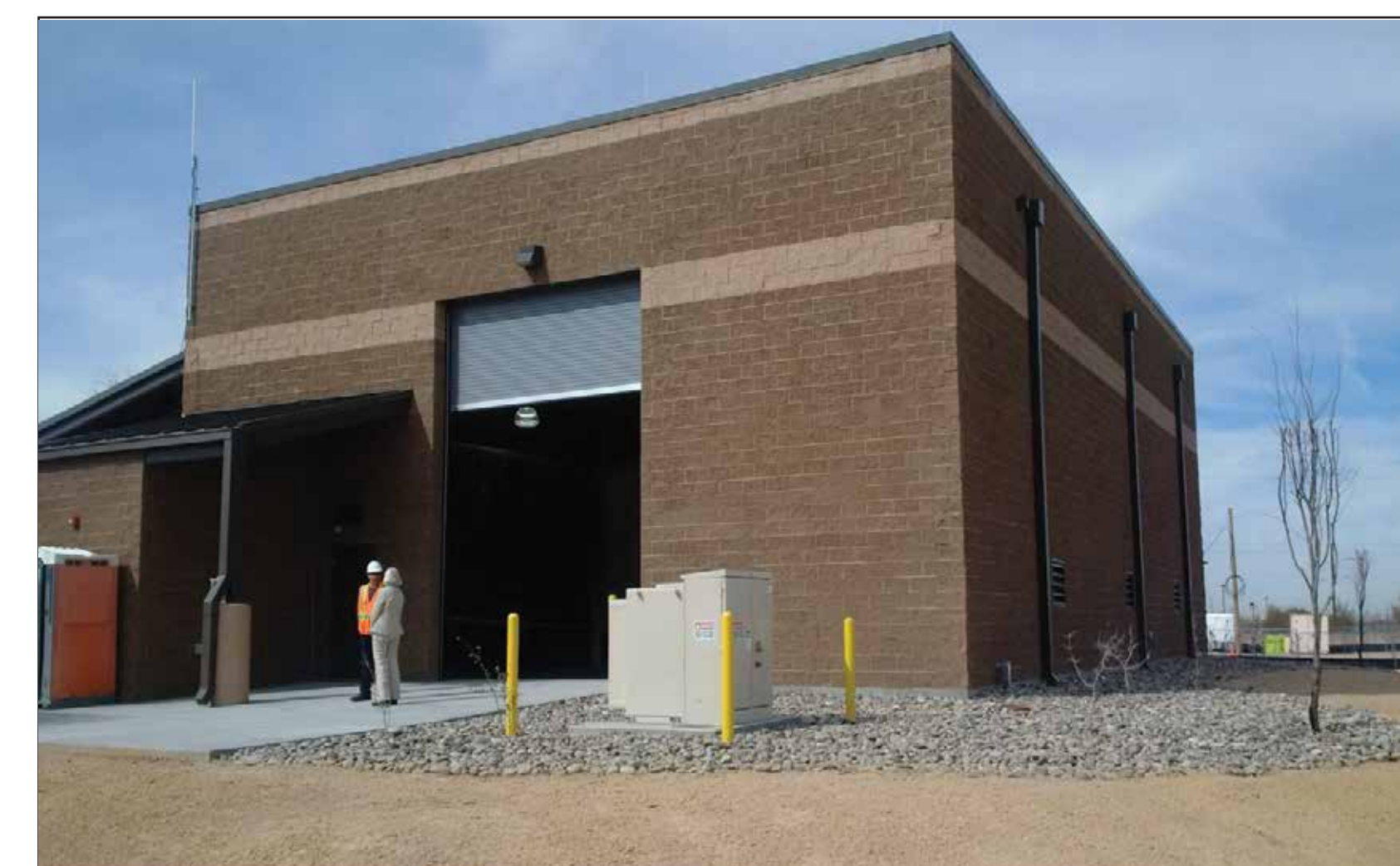
The GWTS began operation on December 31, 2015 with all three extraction wells. The full-scale GWTS consists of an influent holding tank, bag filters, two-20,000 pound vessels containing granular activated carbon, and a treated water storage tank.
