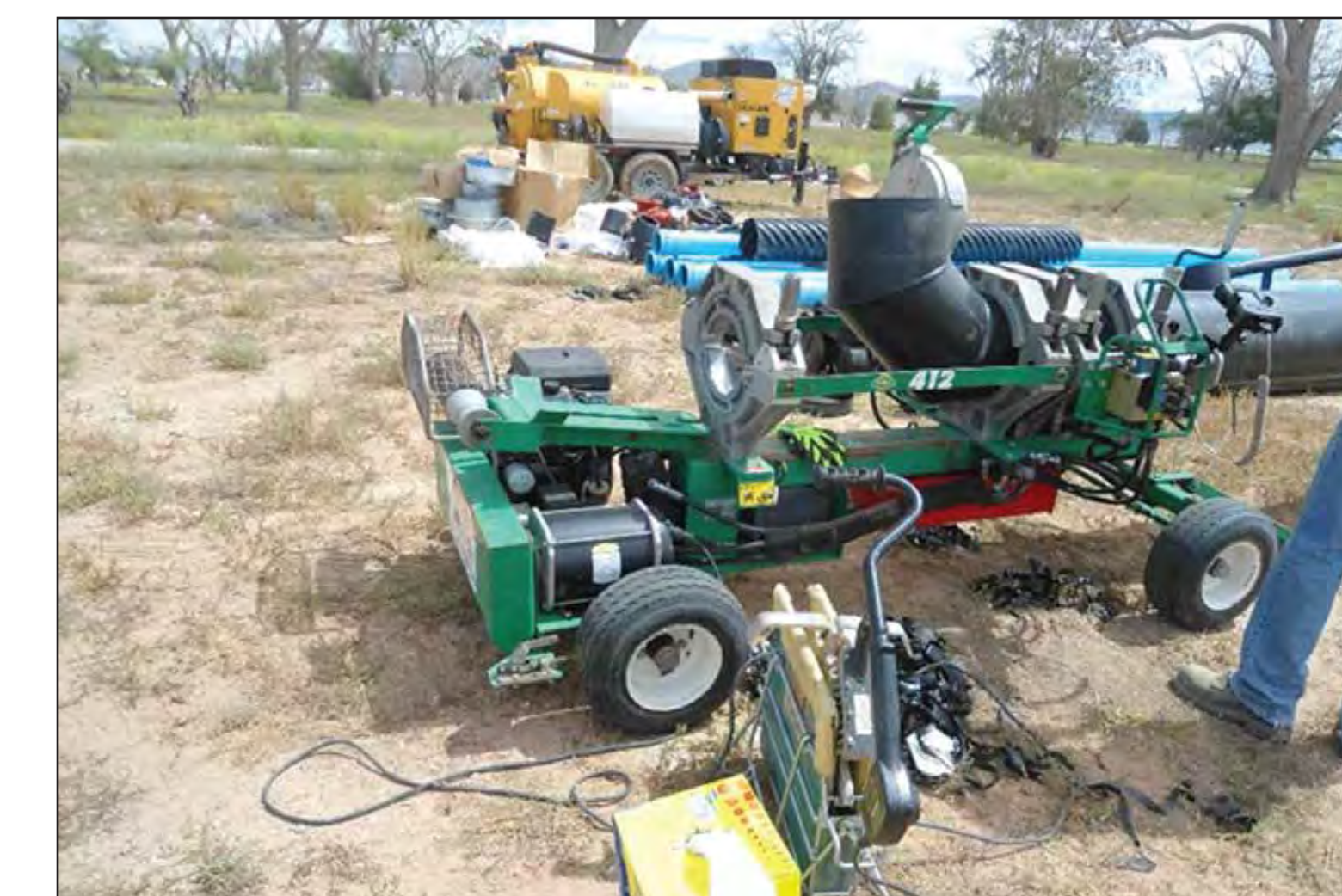
Fusing of the HDPE influent piping. This piping is being installed beneath the ground surface and connects the existing valve vault to the full-scale treatment building.
