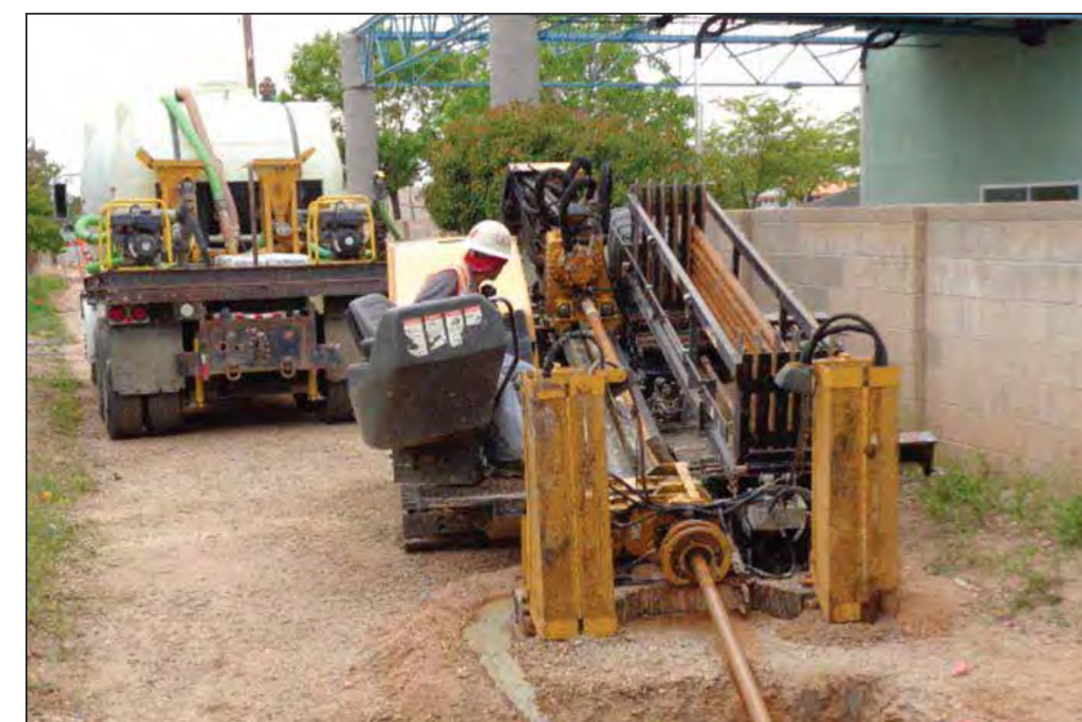
Directional drilling for installation of underground HDPE piping from extraction well KAFB-106228 to Kirtland AFB.
