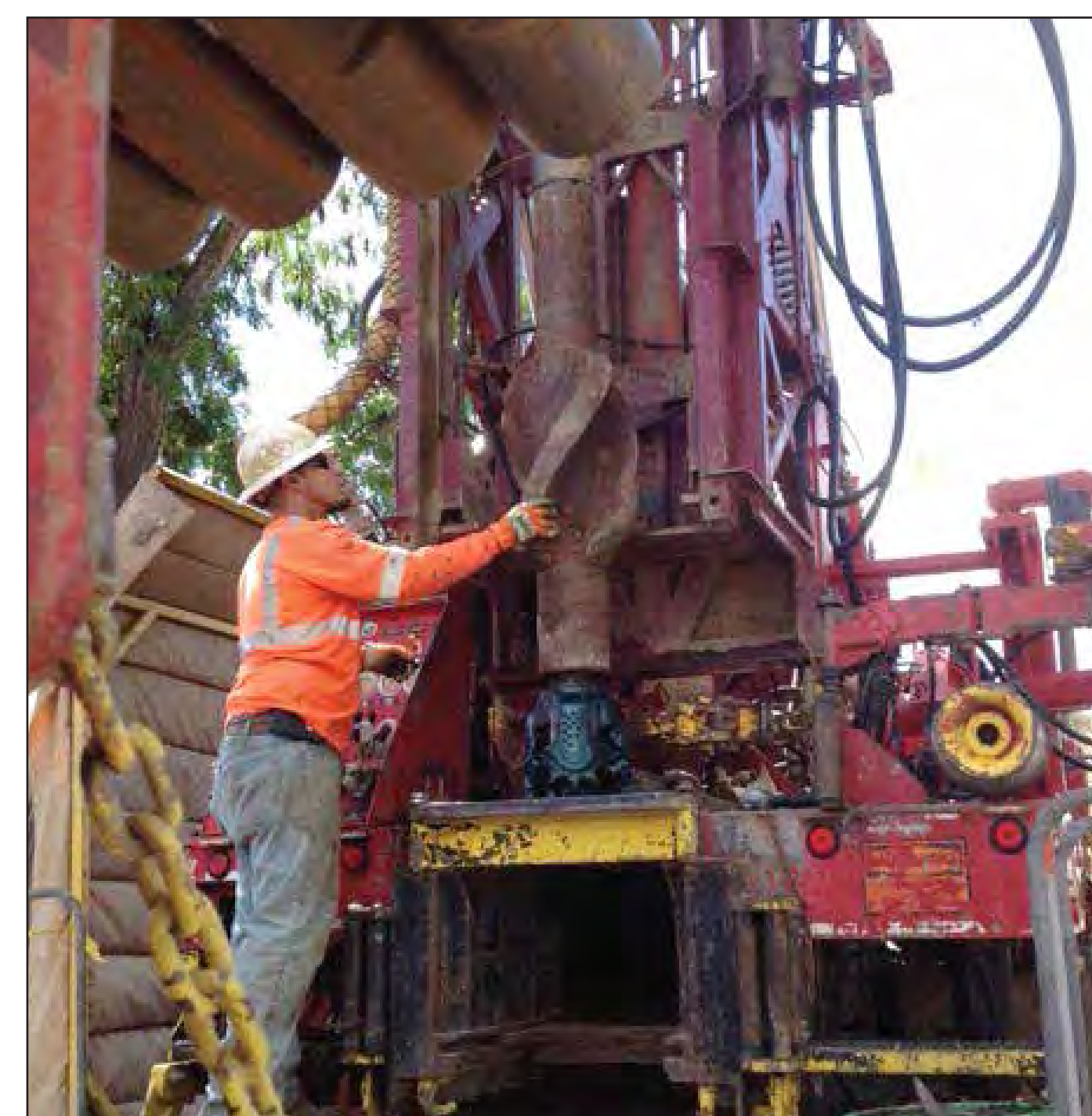
Well 234 Driller inserting bit into well
