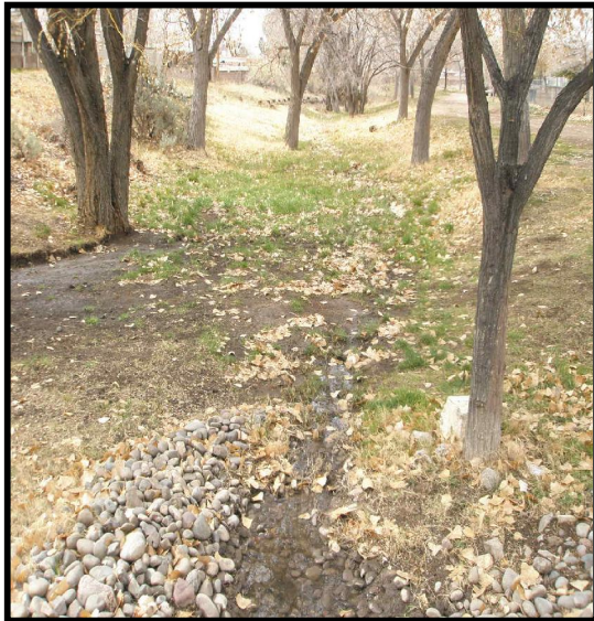
Council Services Tom Bolack Urban Forest Storm Drain
