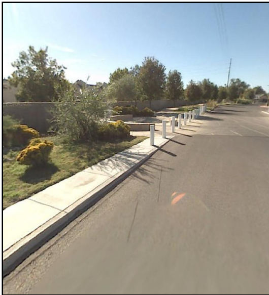
Google Street View Constructed Section of Old Acequia Madre adjacent to Explora Parking Lot
