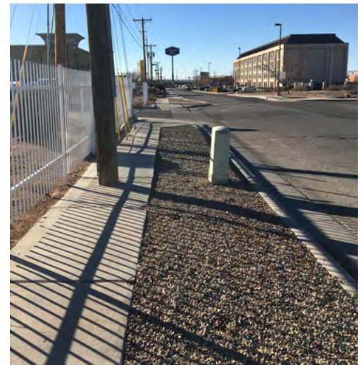
At various locations along Cutler infrastructure is blocking the sidewalk.
