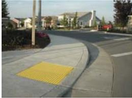
The southeast curb return shows evidence of significant vehicle off-tracking which is a danger to pedestrians in this quadrant of the intersection. Reconstructing this curb return to accommodate a 30-ft radius will allow larger vehicles to navigate the curve without driving through the pedestrian ramp and on the sidewalk.
