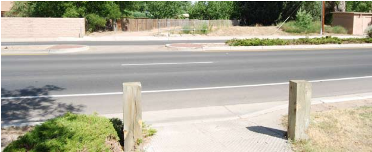
An important trail crossing for equestrians, across Rio Grande Boulevard near the intersection of Headingly Avenue, was identified as a location for improvement. In addition to better markings across the vehicular travel lanes (either as stripping or a different paving material), a wider median is also needed to allow horses to wait as they cross the road.
