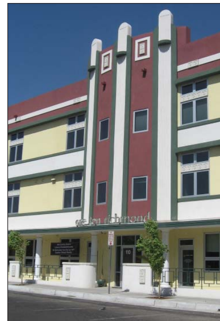
Vertical Mixed Use with office/retail on ground floor and apartments above. Top: Brick Light District on Harvard St. Bottom: 110 Richmond
