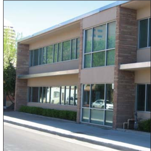
Office Building on Eighth St. - windows cover more than 50% of the ground floor façade and 30% of the second floor façade.
