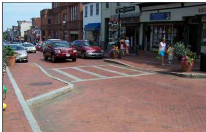
Example of mid-block pedestrian crossing from other communities.
